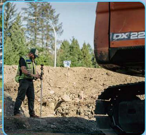
Road construction surveying
